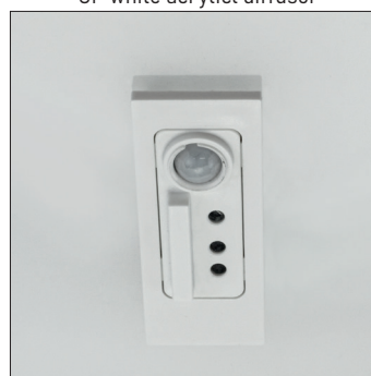
IC daylight&occ sensor
